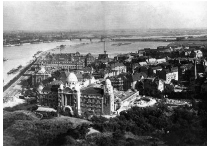
Fig. 3. The embankment at the BME campus [24]
