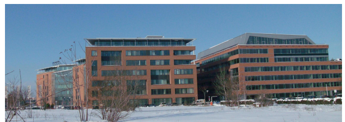
Fig. 5. Buildings D and E of INFOPARK
