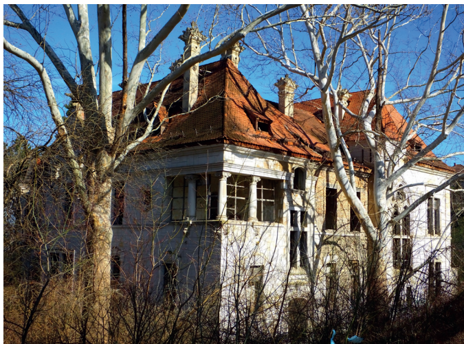
Fig. 2 Spitzer Villa – south façade before roof demolition (Photo: Predrag Komljenović 2016)
