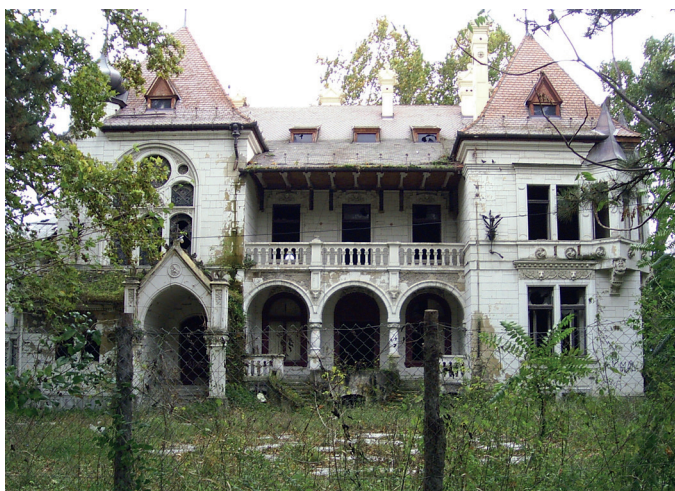
Fig. 3 Spitzer Villa – north façade (Photo: Predrag Komljenović 2004)
