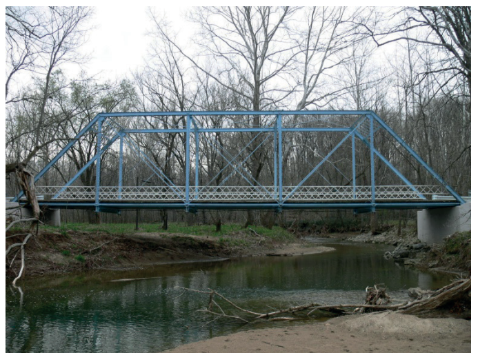
Fig. 6 Hibbs Ford Bridge (89,9 ft), Putnam County, Indiana, 1906. (Photograph by Evan Dillon)
