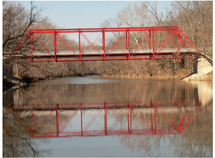
Fig. 4 Lost Bridge (142 ft), Dearborn County Indiana, 1916 (Photograph by Anthony Dillon)
