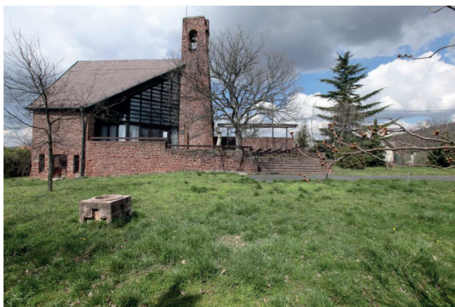
Fig. 3 Révfülöp: outdoor mass of the Church of Saint Joseph the Worker (1978-82).
