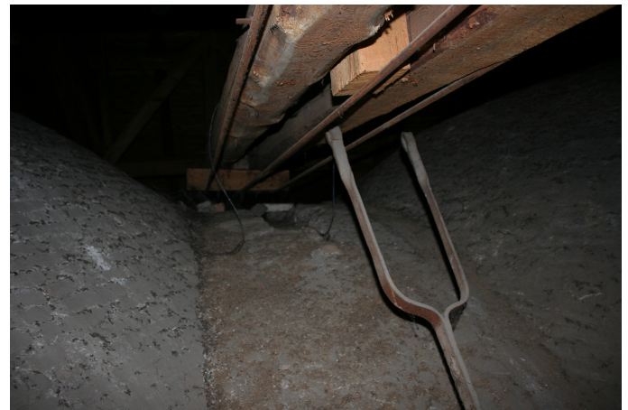
Fig. 6. Disconnected tie-bar over a main arch.
