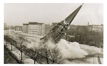
Fig. 4 Radical demolition is a returning issue: detonation of the Versöhnungskirche in Berlin, Germany in 1985 (source: arbetsbok.wordpress.com)
