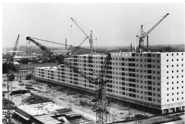
Fig. 3 Óbuda under construction in 1970. Source: Fortepan 74122.
