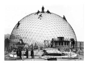
Fig. 12 Steel framework of a 16-m-diameter planetarium test dome, Zeiss Factory Jena, Germany. Design by Walter Bauersfeld and Franz Dischinger, 1922. (Photo: IL Archives Stuttgart, courtesy of Dr. Jürgen Hennike)
