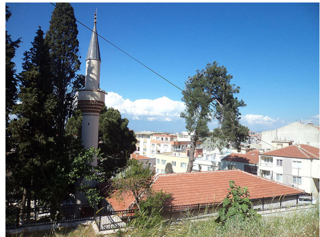
Fig. 6 Haki Baba Mosque and apartment blocks around it - view from the south
