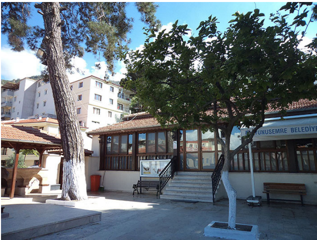
Fig. 8 Haki Baba Mosque, courtyard façade, view from the north
