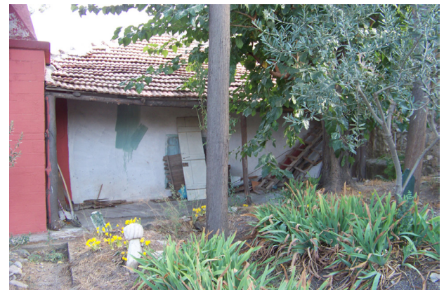
Fig. 4 Timber post remains under the eave, before restoration
