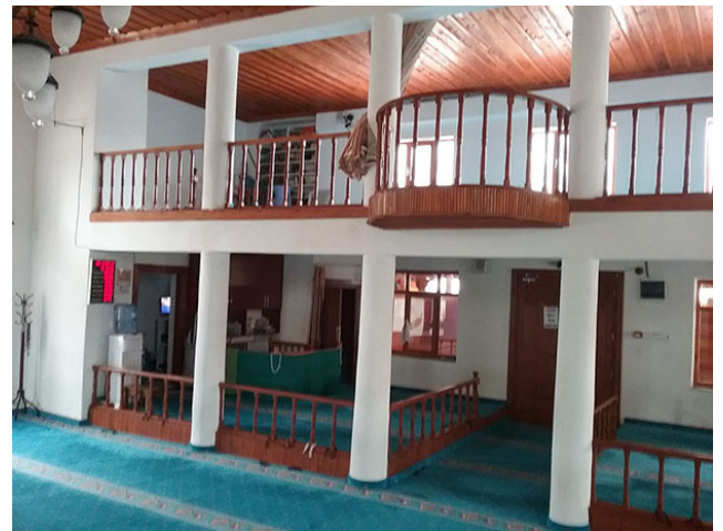
Fig. 14 Spaces and elements at the northern part of the prayer hall, Kabasakal Mosque
