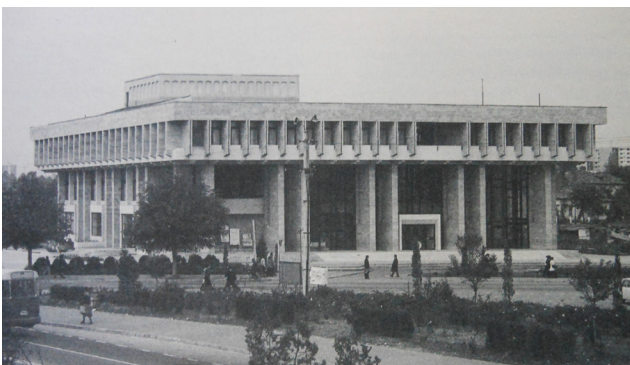
Fig. 4 Echoes of brutalism: the House of Culture of the town of Târgoviște, built 1969–1974 and designed by arch. Nicolae Vlădescu (Tulbure, 2017:p.54).
