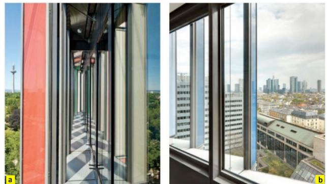
Fig. 18 View into the 700 mm continuous horizontal cavity of the double skin (a) © KfW-Bildarchiv/Thomas Klewar; Double-skin façade viewed from interior showing the colored glass panels that open by pivoting outwards (b) © Jan Bitter.
