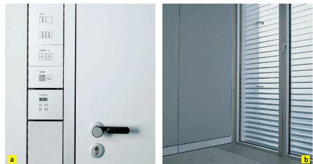
Fig. 8 The control panel next to office doors (a) and an interior view showing perforated aluminum blinds in the façade cavity (b) © Ingenhoven architects.
