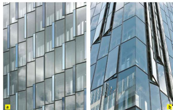
Fig. 22 Façade detail showing flaps letting air into the façade cavity (a); flaps opened at the "tip" to enable through-flow of air (b) © Jan Bitter.
