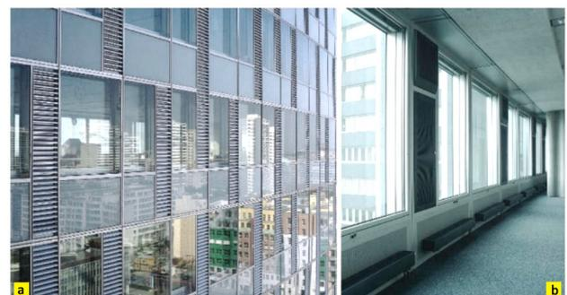
Fig. 11 Louvered air intake openings on the east façade (a); and the inner upper panels which pivot downward for air intake (b) © Annette Kislign.
