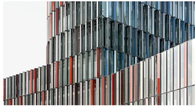
Fig. 17 Sawtooth profile façade with slender colored panels between larger fixed glass panels © Jan Bitter.
