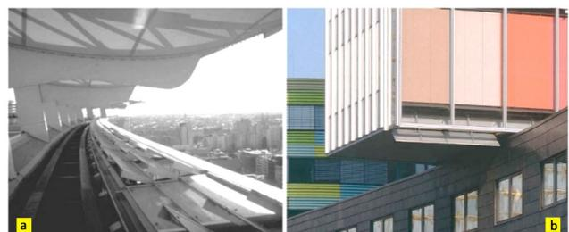
Fig. 14 Dampers located at the top of the thermal flue (a) © Arup and Dampers located at the bottom of the thermal flue (b) © Annette Kising.
