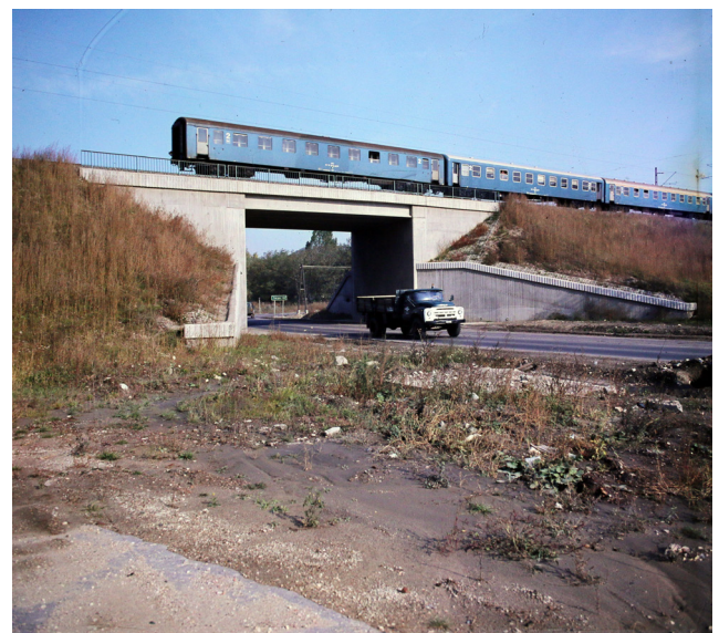
Fig. 1 Railway overpass on the Budapest-Győr line (Source: Fortepan, 1980)
