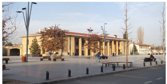
Fig. 15 Gaziantep Train Station, 2017 (Güleç, 2017).
