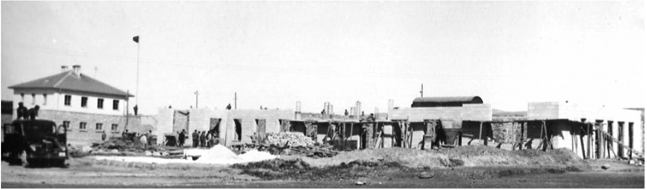
Fig. 13 A view from Gaziantep Train Station worksite- 1950s (Severoğlu, 2018).
