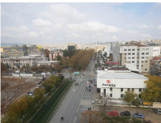
Fig. 10 (up) Old picture of Gaziantep Train Station in the city silhouette (WOW Turkey) (down) Today picture of Gaziantep Train Station from the Station Street looking north, 2018 (Güleç, 2018).
