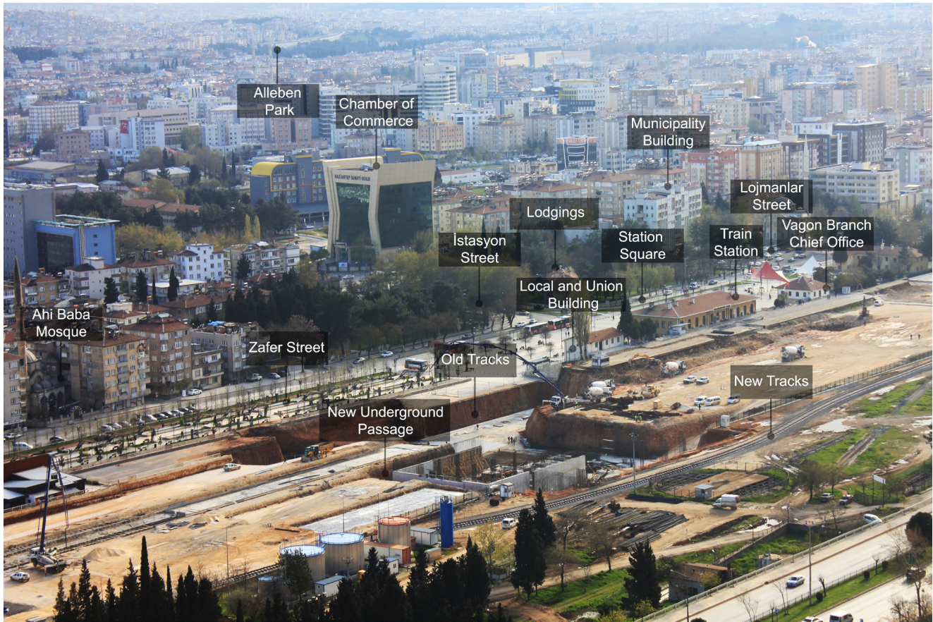
Fig. 17 General View of Gaziantep, showing today's situation of the station and its connection to the city, 2019.
