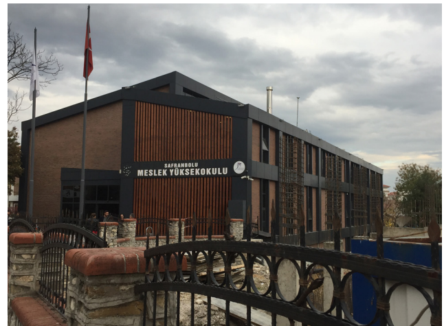
Fig. 1 Safranbolu Vocational High School Building
