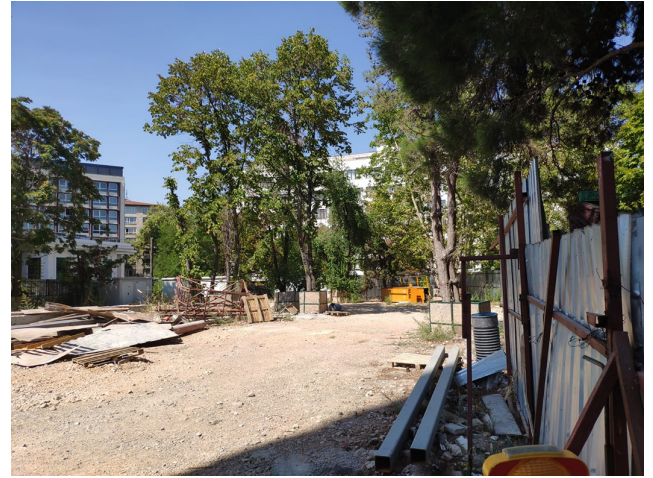
Fig. 27 Construction of the Metro Station in Zafer Park (Akbulut, 2020)
