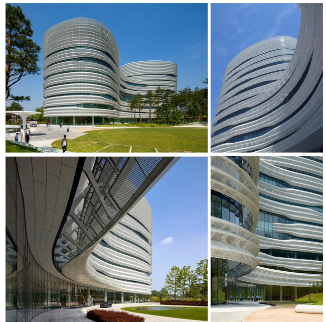
Fig. 4 CJ Blossom Park provides daylight control with moving panels integrated into the facade (A.I.A. Chicago, online)
