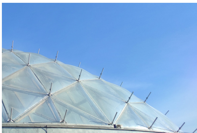
Fig. 1 ETFE covering on Biodóm by Pauliny-Reith & Partners in Budapest (under construction, 2021)
