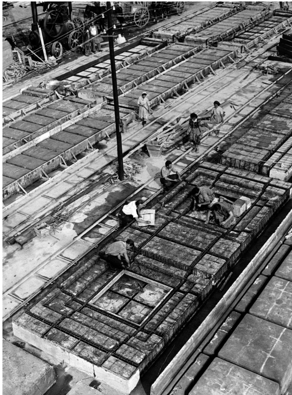
Fig. 1 Prefabrication at Borsod Power Plant, 1952 Anonymous, 1952b)
