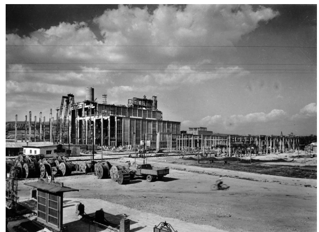
Fig. 3 Overview of the construction site, Inota Power Plant, 1951 (Anonymous, 1951b)
