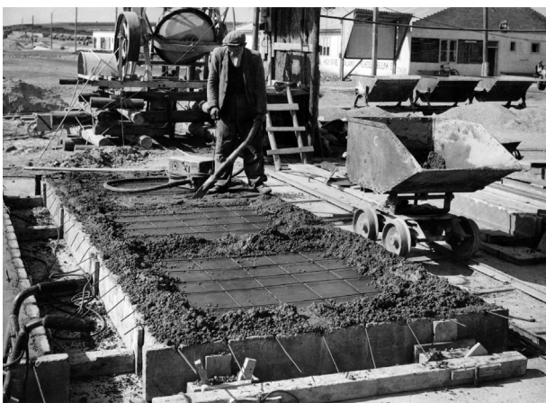
Fig. 2 Manual fabrication of the building of the Inota Power Plant, 1951 (Anonymous, 1951a)
