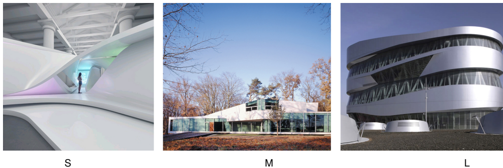
Fig. 11. S - 'The Changing Room', M - Möbius-house, L - Mercedes Museum: Montage: Zoltán Bun
