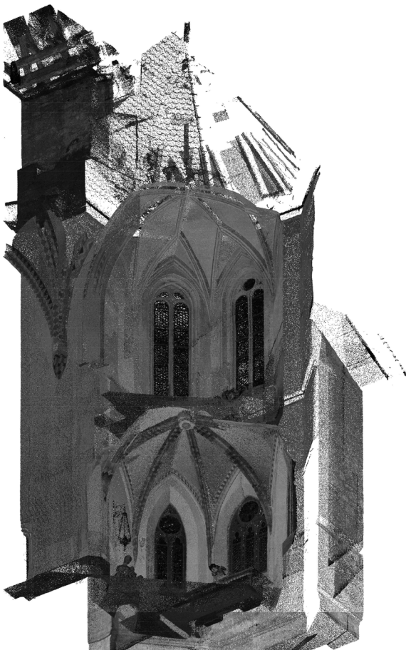
Fig. 1 The picture of the oratorio's point cloud
