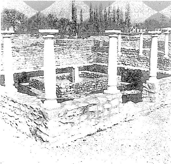
Fig. 4. Budapest – Aquincum. Peristyle court of 'Collegium Inventuti' in the civil town.
