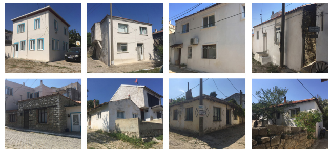
Fig. 6 Examples of traditional buildings in Kilitbahir
