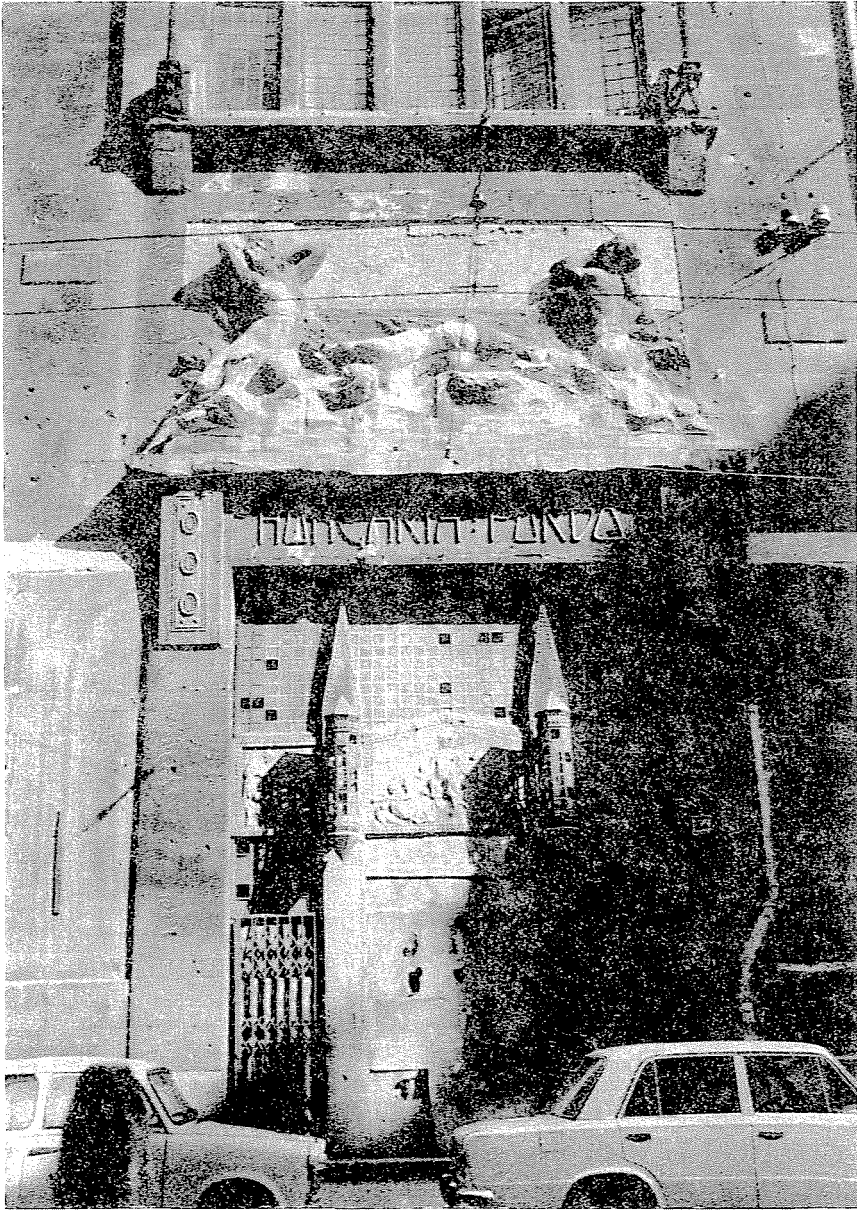
Fig. 12. Swimming pool of Hungaria Bath. Entrance. Actual condition
