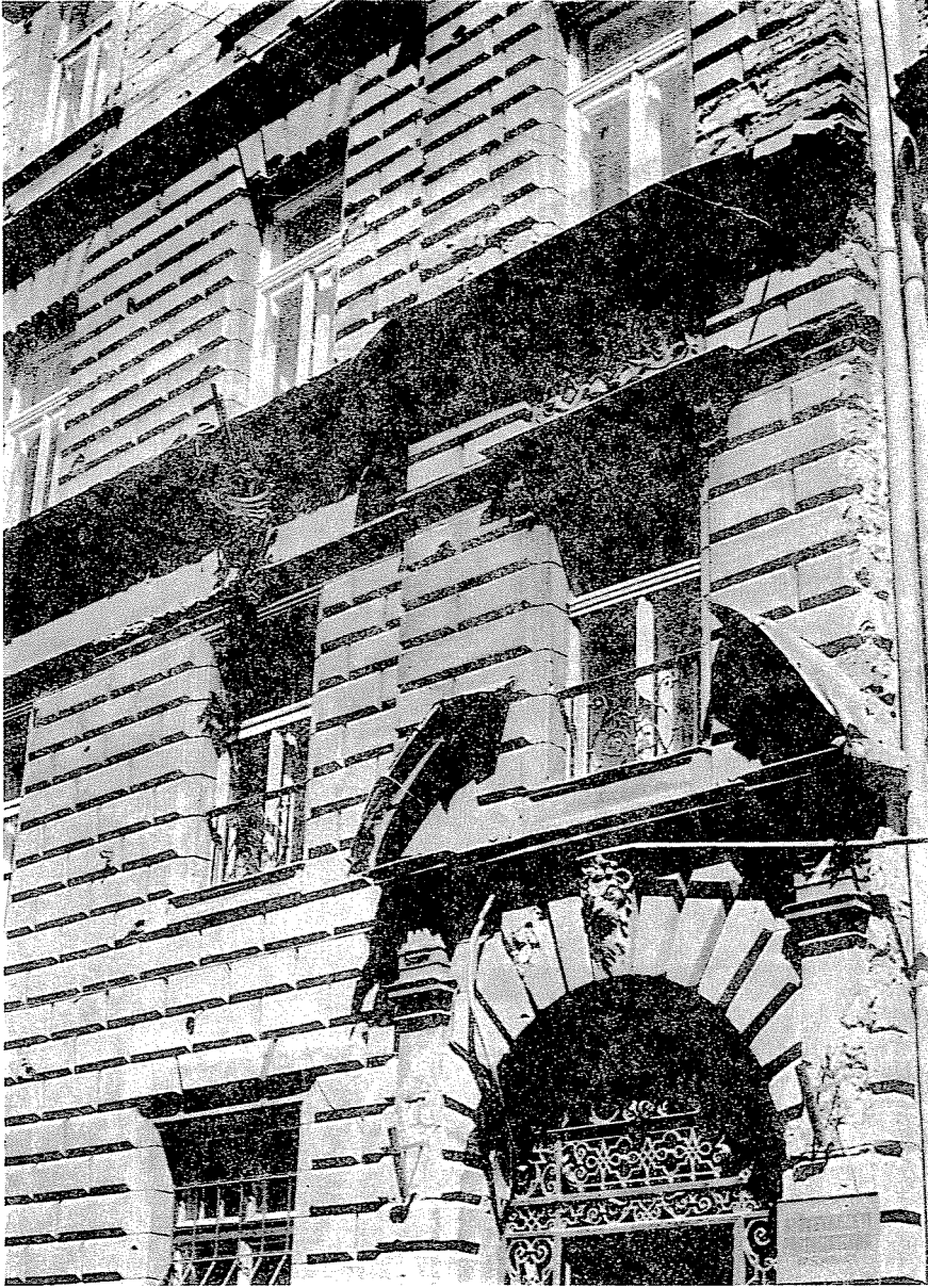
Fig. 10. Hungaria Chalybeate Bath. Remnants of the cornice, and wrought iron flag holder
