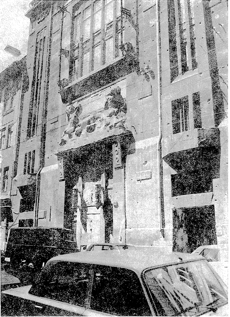
Fig. 11. Swimming pool of Hungaria Bath. Principal façade. Actual condition
