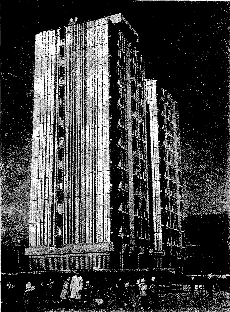
Fig. 3. Large-slab living house, Pécs, 1969. Architect: Ernő Tillai
