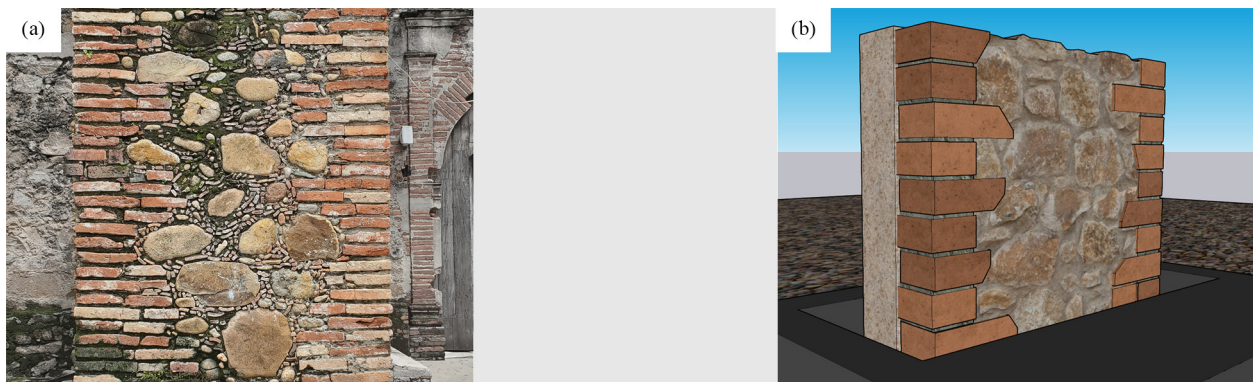
Fig. 2 (a) Typology of masonry walls of the historic temple, (b) Conceptual segment for the elaboration of the wall
