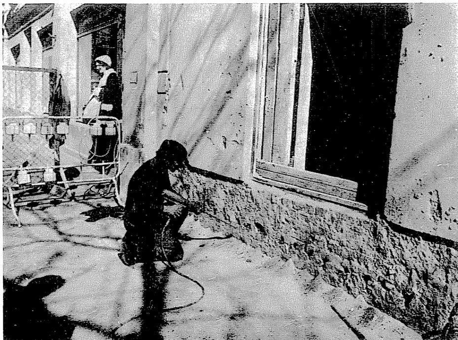
*Fig. 6. Grouting and borehole sealing*
