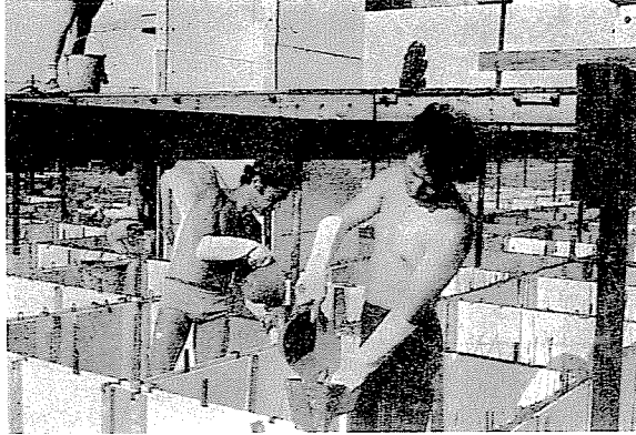
Photo 22. Concreting. The units are clipped to the "lugs" of the timber auxiliary structure. Moisture absorption by gypsum immediately stiffens the concrete, eliminating thereby the hydrostatic pressure
