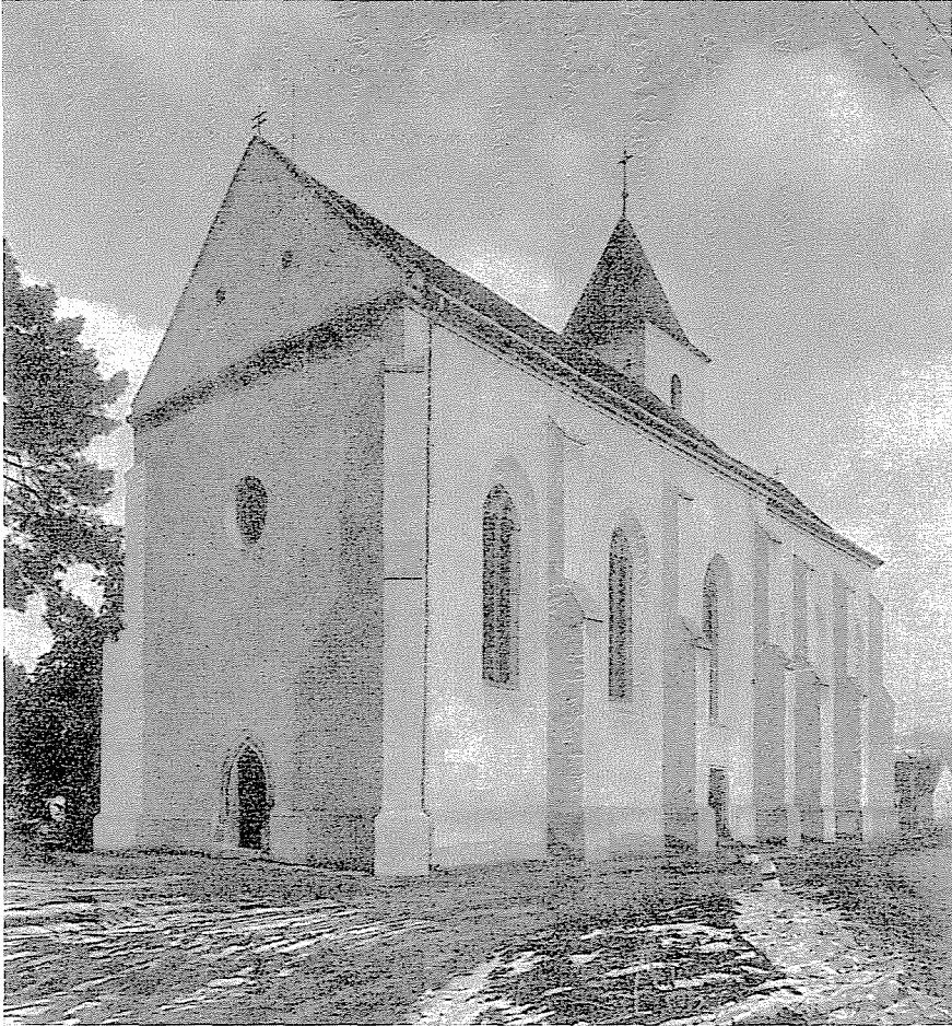
Fig. 5. Gothic church at Köröshegy (Hungary) reconstructed by the author 1968 to 1970, using rendering admixed with Bayer F powder on W and N footings. Buttriss on the SW corner exhibits a marked difference between conventional and experimental rendering
