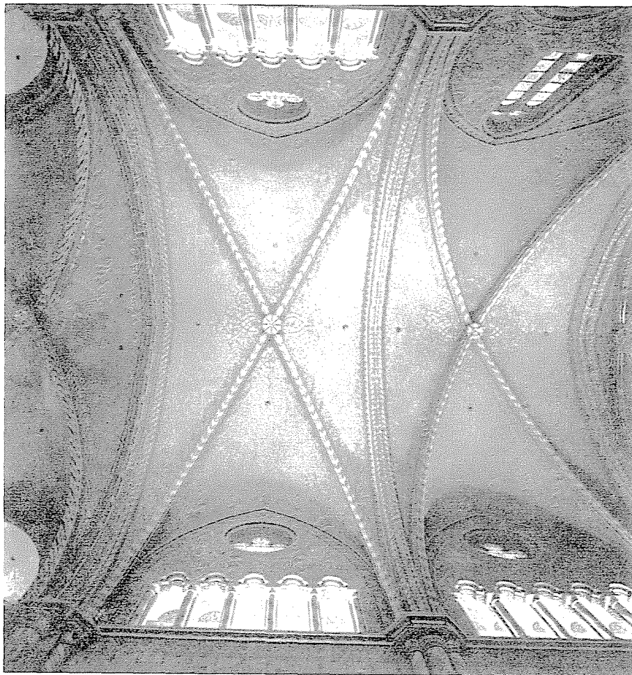
Fig. 2. Mathias Church, Budapest. In spite of heavy soaking of the vault above the sanctuary after reconstruction, the Sikurite plastering prevented any but slight damage. A perfectly aerating plastering could prevent even this damage. (Interior reconstruction 1966 to 1970 by the author)
