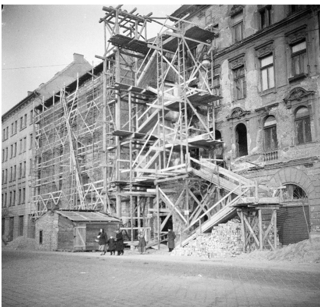
Fig. 3 Restoration works in 1954 (Keveházi, 1954)
