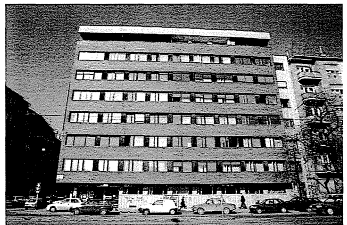
Fig. 6. Apartment house. Fehérvári út 17.
