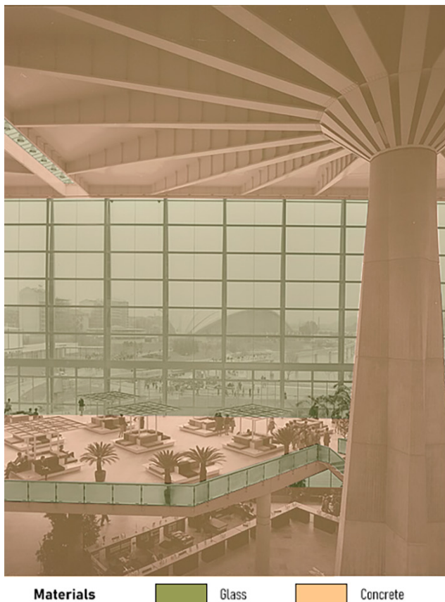
Fig. 4 Materiality of the building's structure (Edited by the author based on Monti (1961b, CC BY-SA 4.0))
