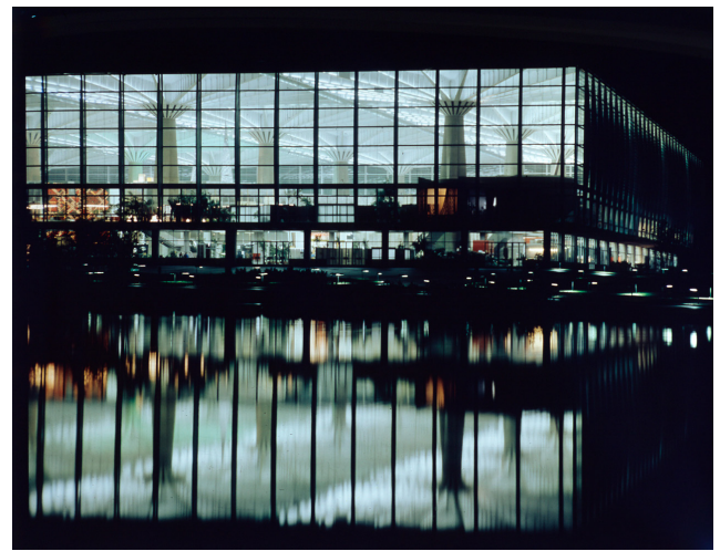
Fig. 5 Palazzo del Lavoro: Column system seen from outside (Edited by the author based on Monti (1961c, CC BY-SA 4.0))
