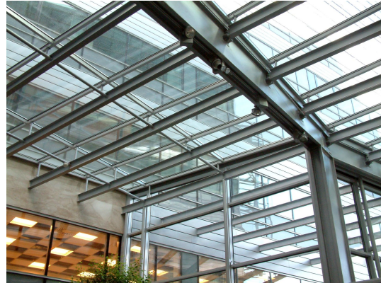
Fig. 2. Loadbearing structure + glazing bar construction roof.
