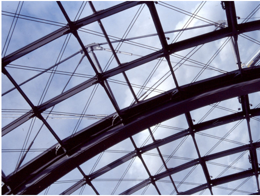
Fig. 3. Lattice shell construction.
