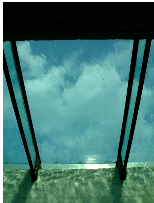
Fig. 5. Glass fields supported by glass beams.
