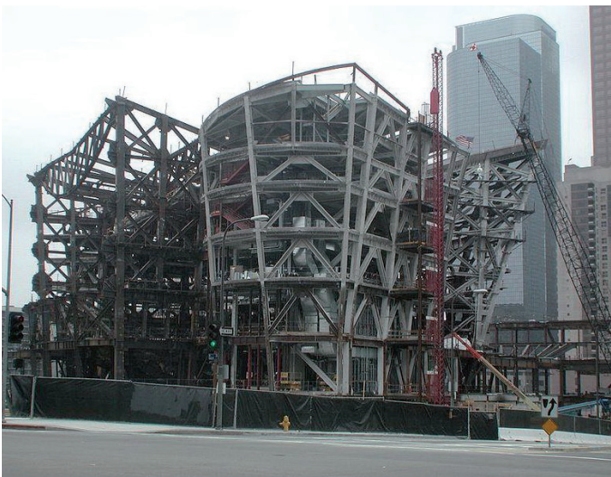
Fig. 5. Walt Disney Concert Hall - Load bearing construction [resource: wikipedia]
