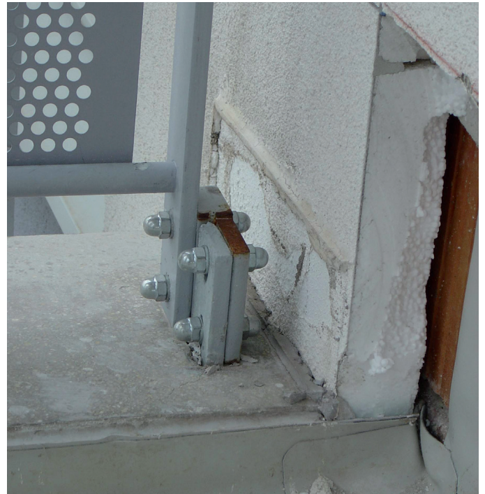
Fig. 18. Damaged thermal insulation on elevation
