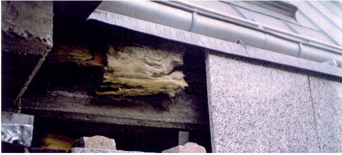
Fig. 16. Damaged thermal insulation on roof edge
