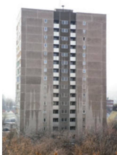
Fig. 7. Block of flats in Kelenföld (moisture can be seen on a large area, covering entire panels of the building).
