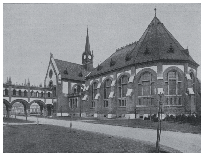
Fig. 12. The Library Building from north in 1909. (After Balogh, R. [3] [6, p. 490] [12, p. 20] [25, pp. 232-233])
