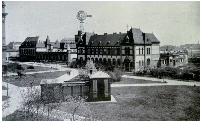
Fig. 6. The MM-MG and MT buildings from west, 1920s. (After [14, vol. 7. p. 1632] [25, pp. 230-231])
