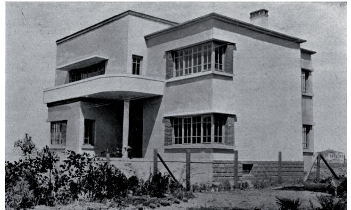
Fig. 11 Şevket Bey House, Mimar, 1933-28.
