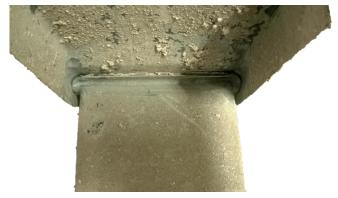
Fig. 3 Connection failure of encased elements
