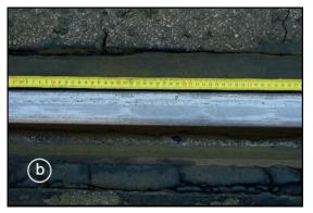
Fig. 10 Vertical wear of rail head. The wheel flange running on the bottom of groove of the grooved rail. Long-wavelength rail corrugation on rail head. (See Fig. 6d. outstanding values at the section (b))
