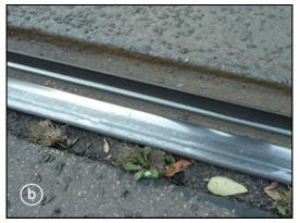
**Fig. 8** Sinked rail and laterally weared rail groveed head (See Fig. 5c. outstanding values at the section of (b) between 55–63 s)
