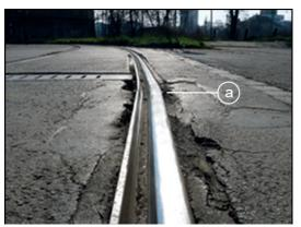
Fig. 7 Lateral misalignment on the outer rail (right side) in curved segment (See Fig. 5c. outstanding values at the place of (a) about 40 s)
