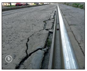
Fig. 11 On the straight segment 3, the sinked rail and fragmented pavement (See Fig. 6d. outstanding values at the section (b) between 58–68 s )
