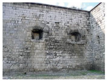
Fig. 1 Strongly weathered porous limestone wall, Citadella fortress (Budapest). Note the black crust formation and scaling crusts on the wall.
