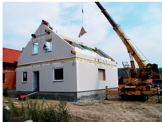
Fig. 3 Construction of a panel construction system [21].
