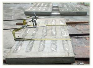
Fig. 5 AAC-concrete lightweight precast ferrocement composite floor slab
