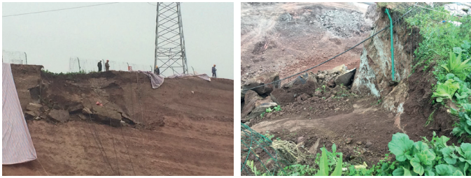
Fig. 18 Wedge failure during excavation
