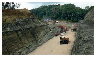
Fig. 7 The steepest and highest benches at the base of the cutting in sandstones and tuffs, correspond to higher UCS, higher  $V_p$  and higher Q-values, with inter-correlations as shown.
