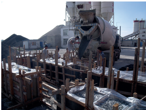
(a) Casting concrete
