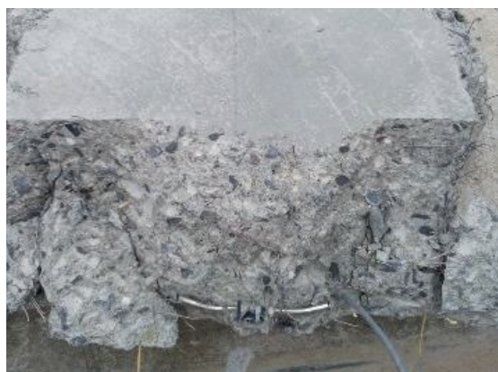
Fig. 16 The EDS_20V_E strain gages used for the measurement, a damaged strain gage after the completion of measurement
