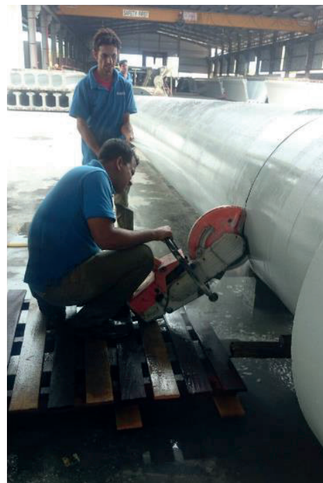
Fig. 8 Cutting the CFBC with segments sections from the real tower
