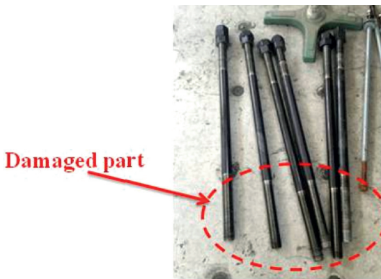
Fig. 16 Loosened bolts in the foundation
