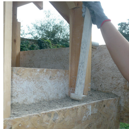
Fig. 3 Direction of compaction of the mixture in a wall formwork
