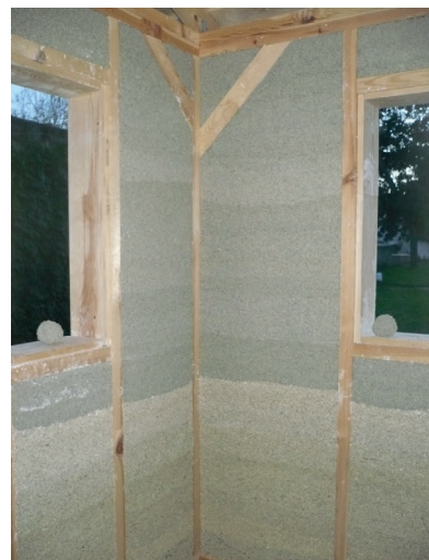
Fig. 5 Hemp-lime composite between timber studs on the inner side of the external wall
