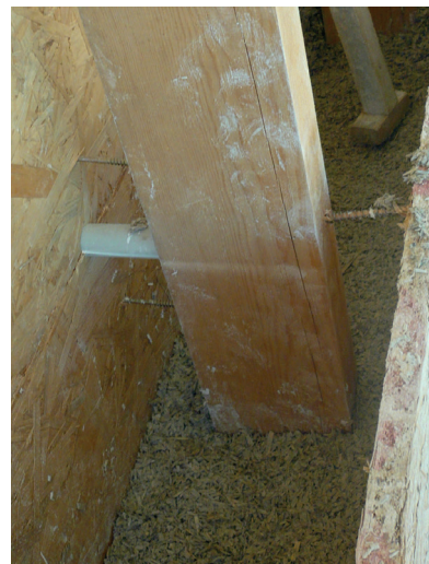
Fig. 4 Hemp-lime composite between timber studs in the middle of a wall
