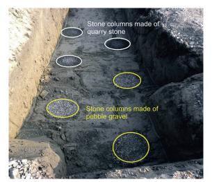
Fig. 1 Stone columns in the area tested
