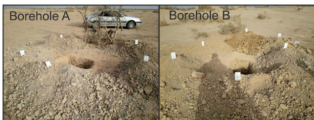
Fig. 2 A view of the boreholes A and B
