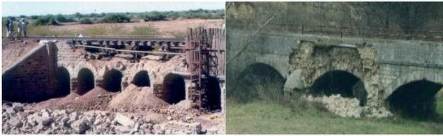
Fig. 2 A railroad bridge damaged in India 2001 Bhurj earthquake [1]
